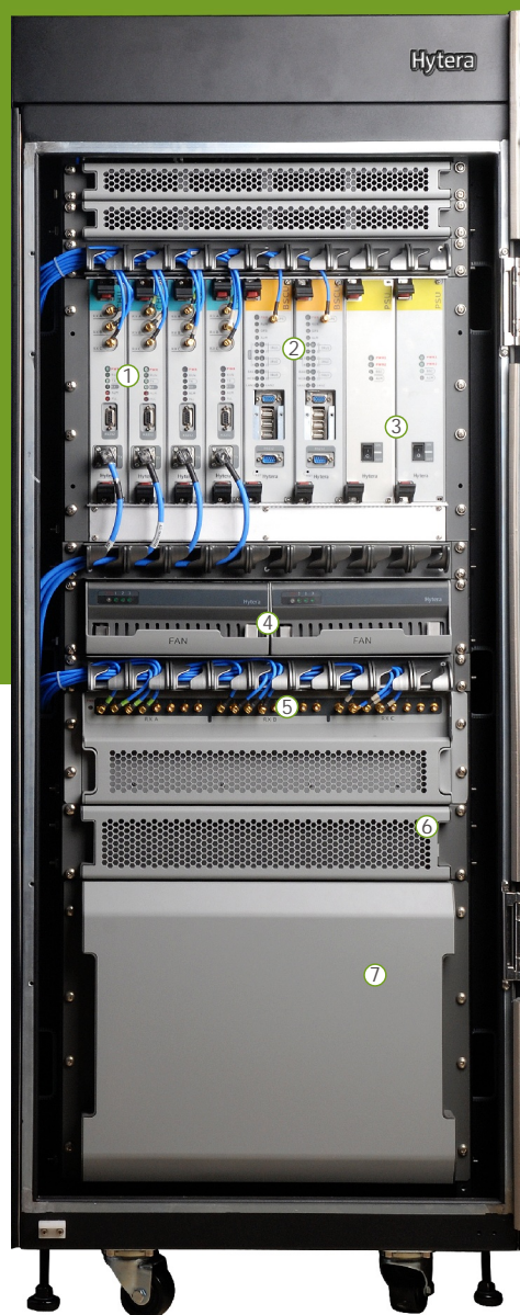
DMR digital trunking base station
